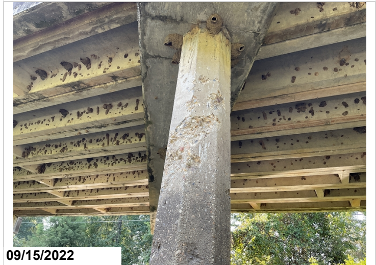
Bent 4 pile 5 spalls from gun shots
